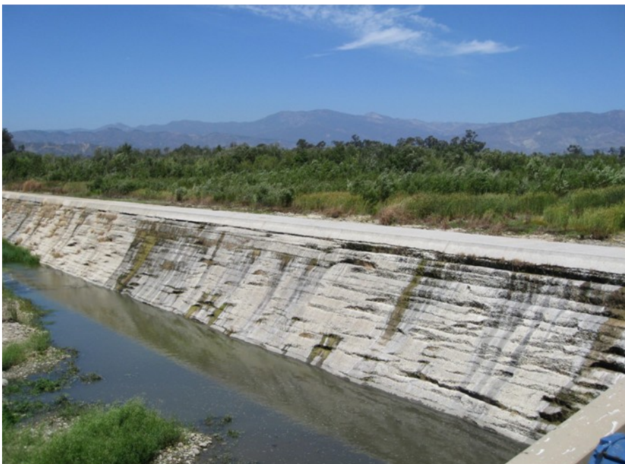
The face of the Freeman Diversion Dam at Saticoy
