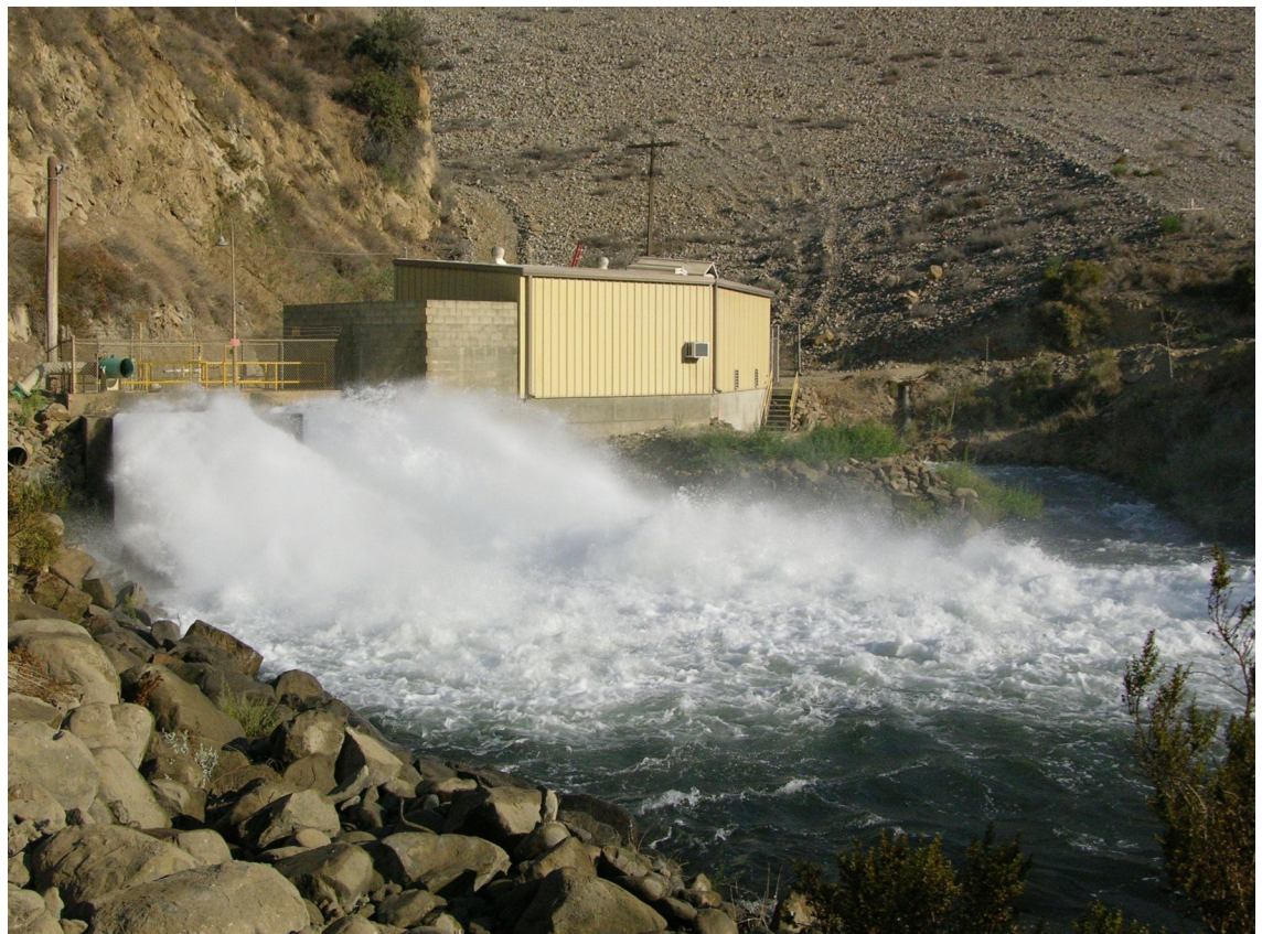
Water Conservation Release from Santa Felicia Dam in 2007
