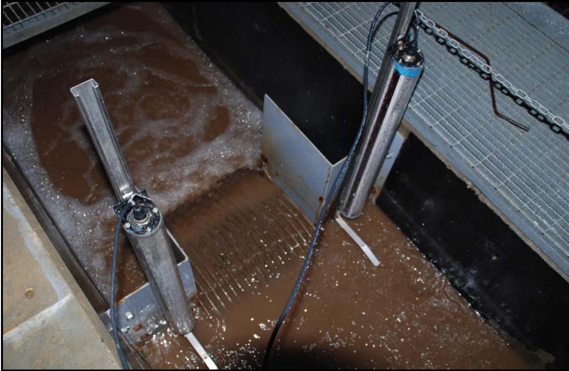
Photo 3 - False weir and infrared fish counter, Freeman Diversion Fish Ladder
