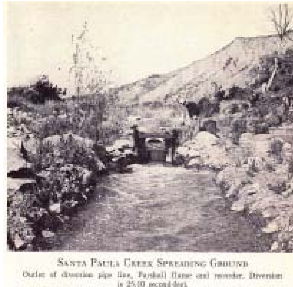
Figure 7. Diversion to spreading grounds in Santa Paula around 1930. This facility was abandoned in 1942.
