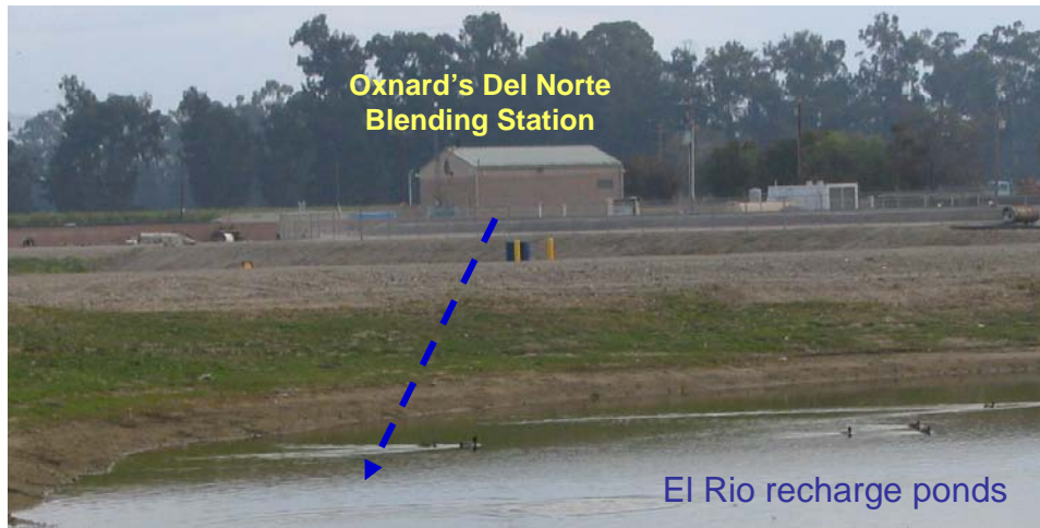
Figure 10. An emergency interconnection between Oxnard's Del Norte Blending Station and United's El Rio spreading grounds will improve reliability during a water quality emergency.
