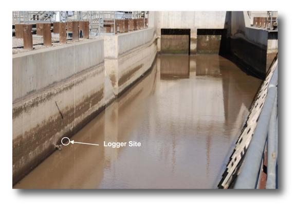
Photo 15 – Fish Screen Bay Water Temperature Monitoring Site
