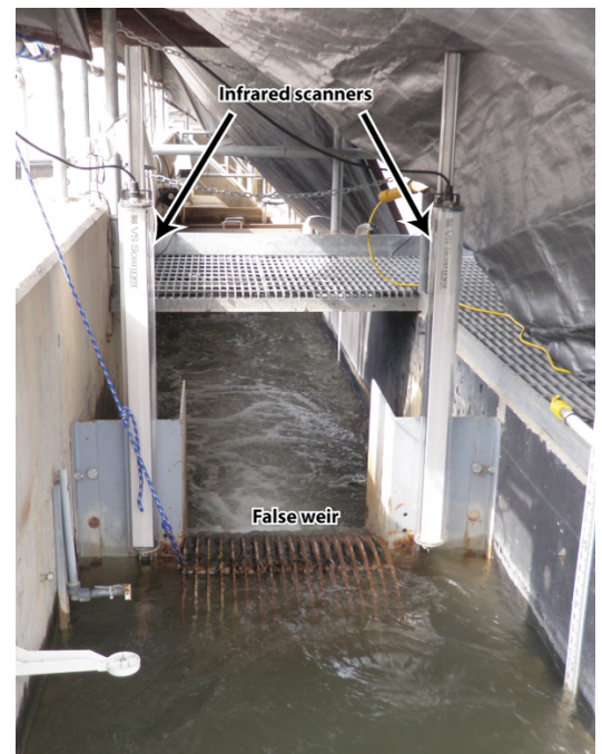
Figure 2. Denil fish ladder false weir
