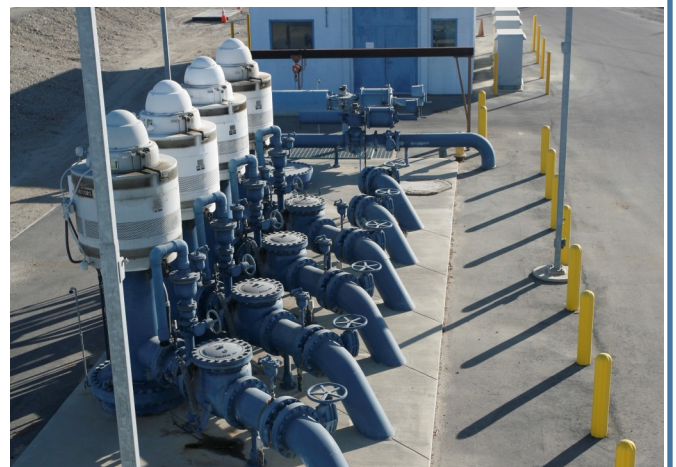
OH Booster Plant and variable frequency drive.
