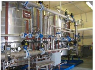
Figure 15 - Infilco Degremont (now Suez) FERAZUR<sup>®</sup> and MANGAZUR<sup>®</sup> System
