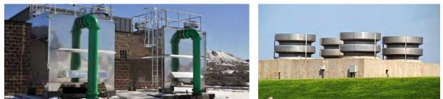
Figure 11 - Induced Draft Aerator (left) and Cascade Aerator (right) (WesTech Engineering)
