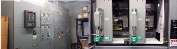
Figure 25 - Existing MCC-C (Left) and Spare Circuit Breaker (Right)
