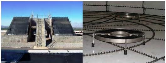
Figure 10 - Cascading aerator at Lake Havasu (left) and in-tank aerator offered by EP Aeration (right)
