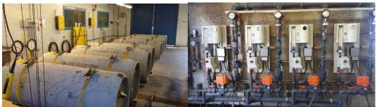
Figure 22 - Existing Chlorine Gas Cylinders (Left) and Pumps (Right)
