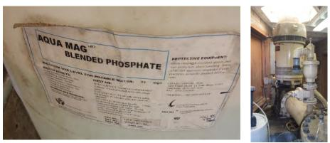
Figure 9 - Well No. 14 and use of AQUA MAG Blending Phosphate
