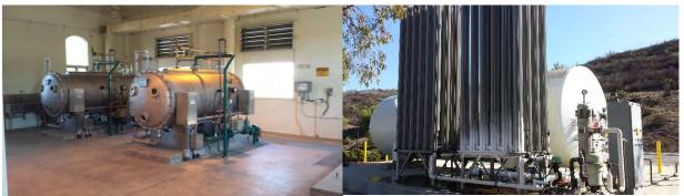
Figure 12 - Ozone generator (left) and pure oxygen storage (right) at CMWD's Lake Bard Treatment Plant
