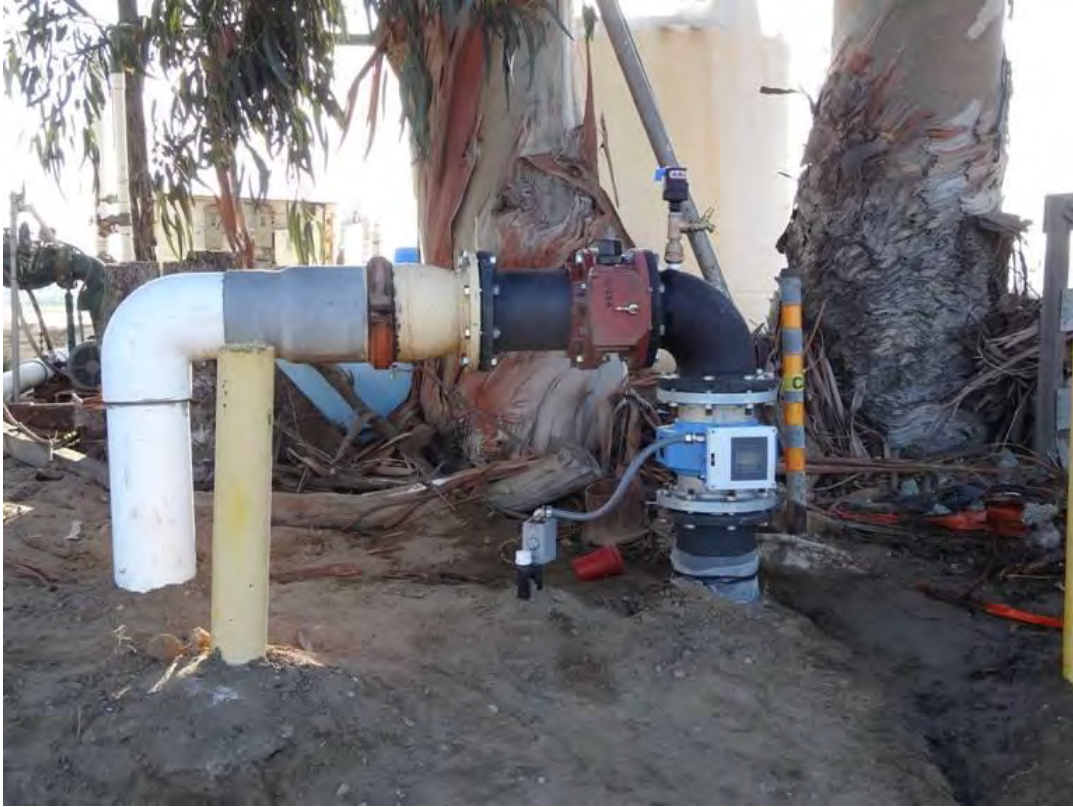
Figure 3 – O&M Staff completed the installation of a new meter at PTP Turnout No. 133
