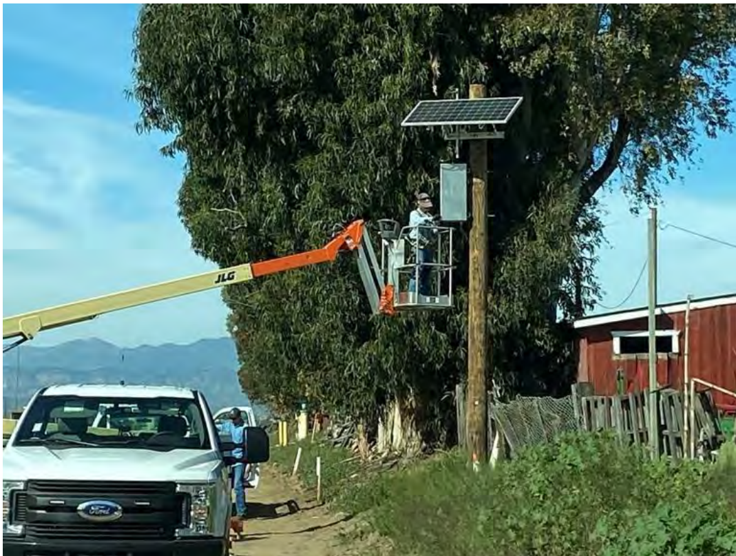
Figure 4 – O&M Staff installing solar power wood utility pole at PTP Turnout No. 133
