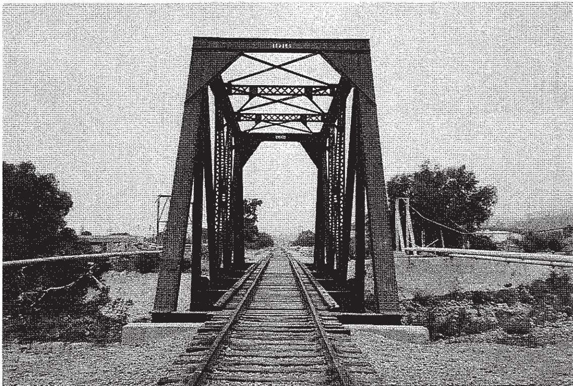
Photo. No. 14. This view shows the three pipelines that need to be relocated. Texaco's 8-inch crude oil pipeline is located to the left (downstream) of the bridge. The first pipeline to the right (upstream) of the bridge is the 10-inch gas line owned by Shell Pipe Line Corporation and next to it is the 8-inch crude oil pipeline owned by Unocal. (June 1994)
