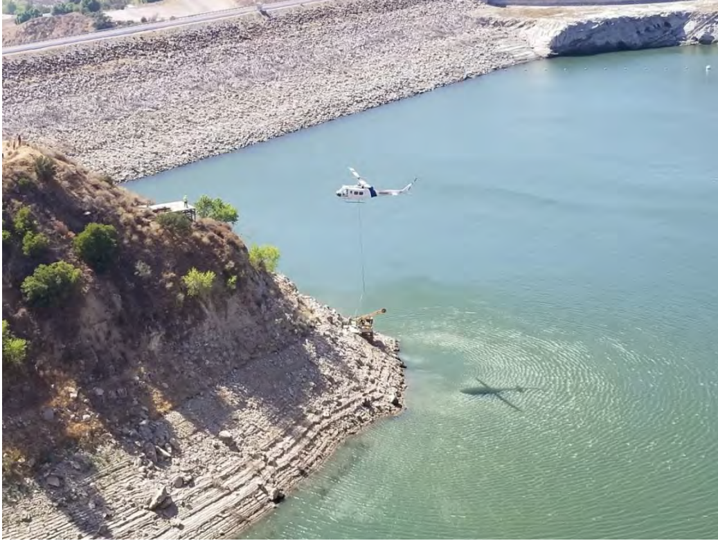
Figure 3 – Mobilization of equipment and drilling rig for Boring B403.
