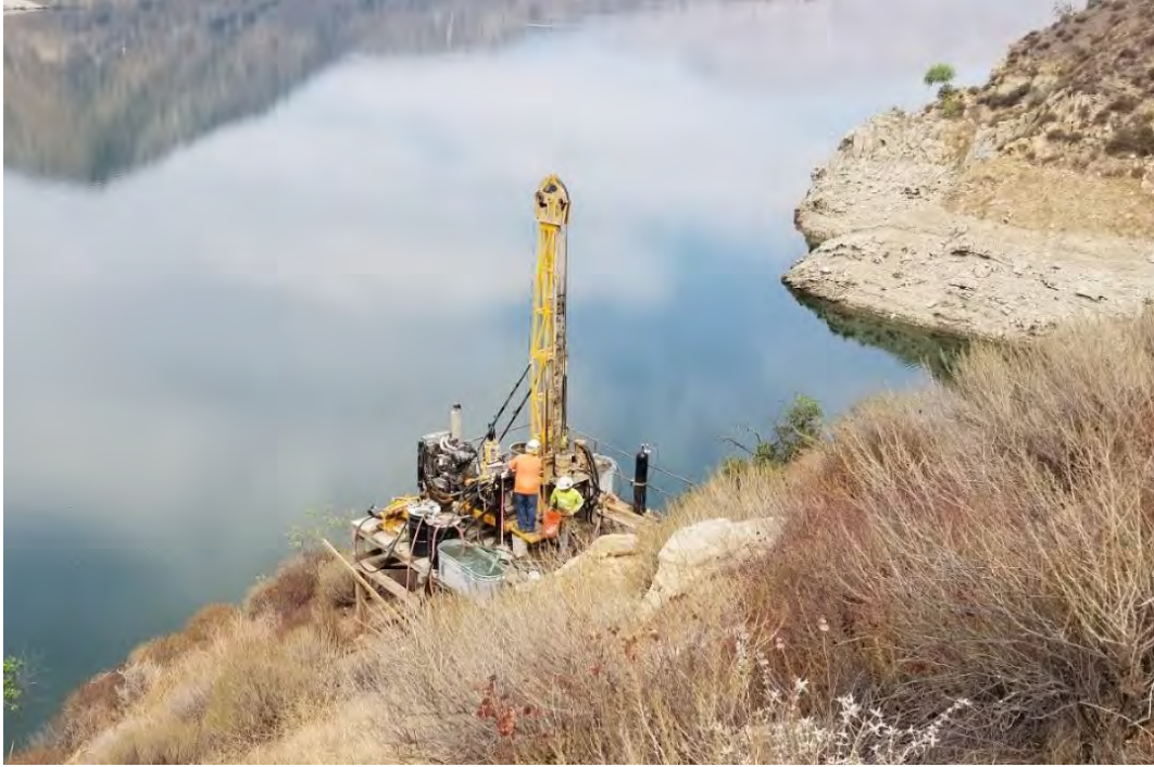
Figure 1 –Drilling operations at Boring B402 from a Platform built on the East Abutment of SFD during the 2020 Drilling Program Plan.
