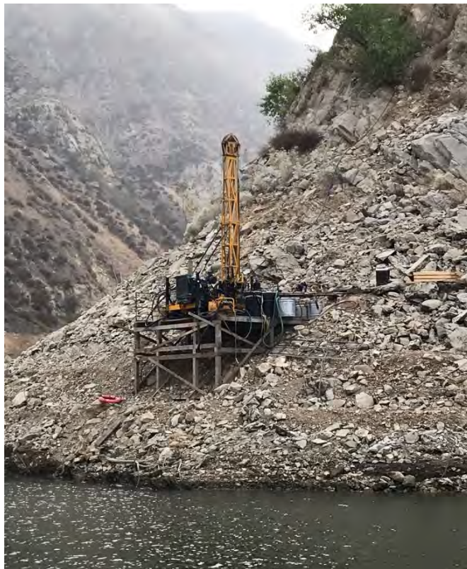
Figure 2 – Platform and Drilling Operations at Boring B403 located on the SFD East Abutment.
