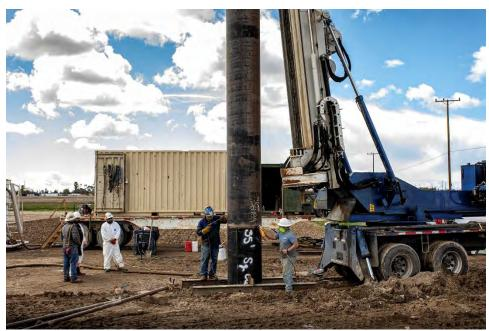
Figure 4 – OH Well Replacement Project – Installation of the Conductor Pipe
