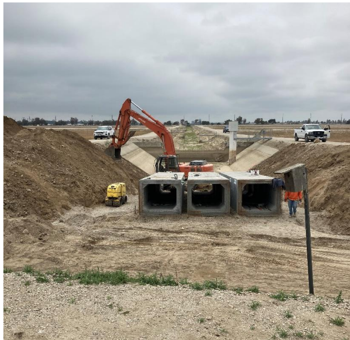
Figure 3 – Grand Canal Project – RCB Installation
