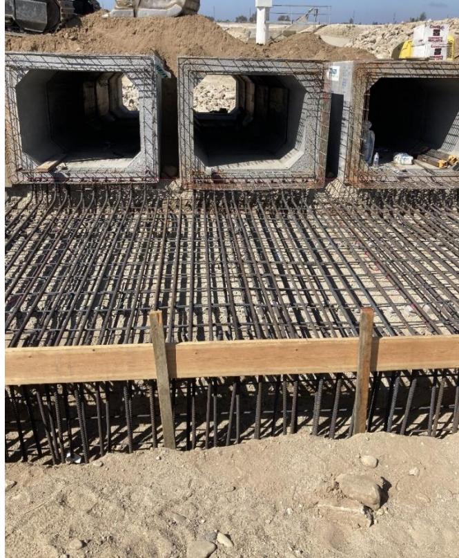
Figure 4 – Grand Canal Project – Intake Structure Rebar
