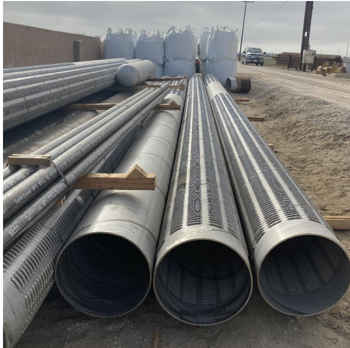
Figure 6 – OH Well Replacement Project – Well Casing Prior to Installation
