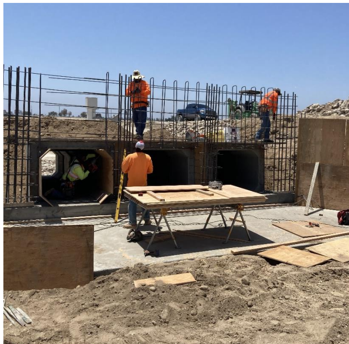
Figure 5 – Grand Canal Project – Intake Headwall Rebar
