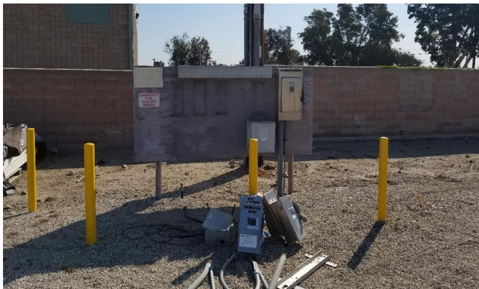
Figure 8 – OH System Backup Generator Project – Existing Electrical Panels Removal
