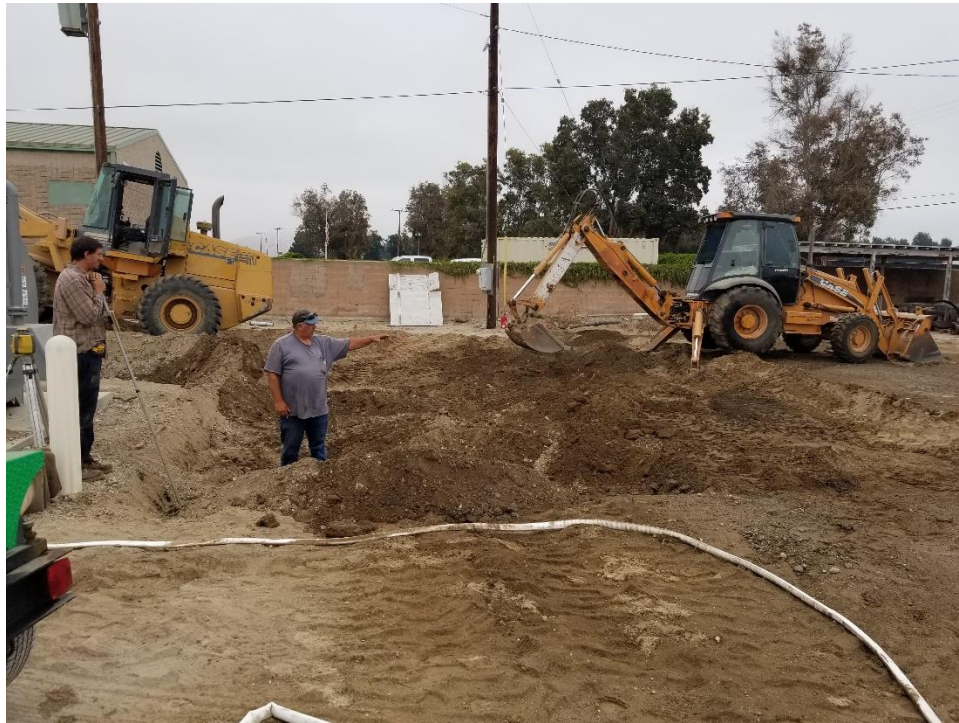
Figure 10 – OH System Backup Generator Project – New Generator Pad Over-Excavation
