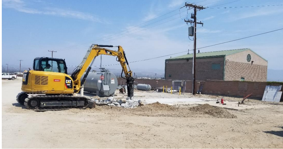
Figure 9 – OH System Backup Generator Project – Existing Generator Pad Demolition
