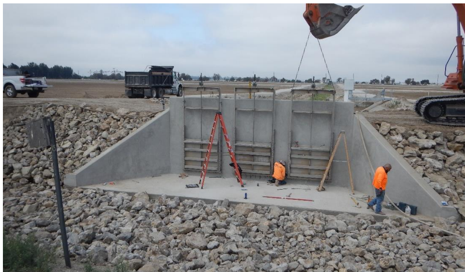
Figure 4 – Grand Canal Headworks Gate Installation
