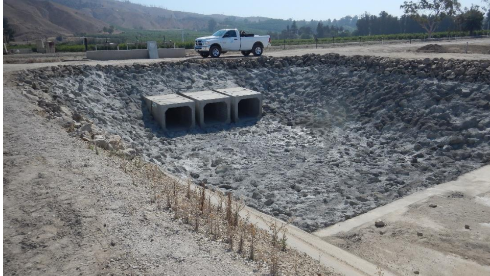
Figure 5 – Grand Canal Headworks Grouted Rip Rap
