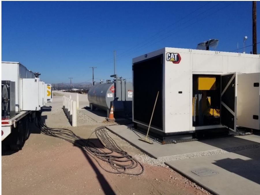
Figure 8 OH System Backup Generator Project – New Generator Load Bank Testing
