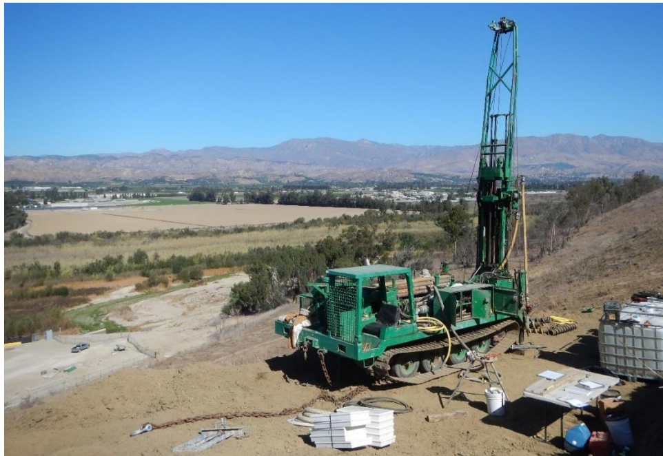
Figure 2 Freeman Diversion Rehabilitation/Fish Passage Facility – Geotechnical Investigation - Installation of the Inclinometer on hillside above Freeman
