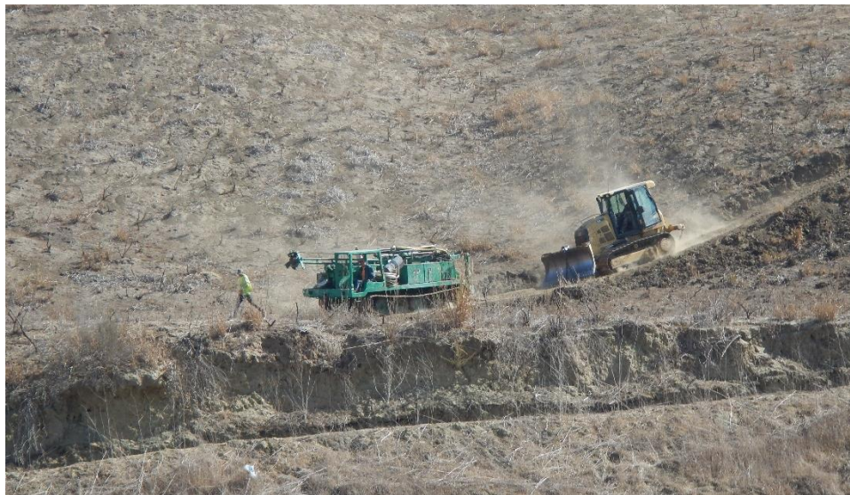
Figure 4 Freeman Diversion Rehabilitation/Fish Passage Facility Geotechnical Investigation - Installation of the Inclinometer (Waking the Drill Rig downhill upon work completion)
