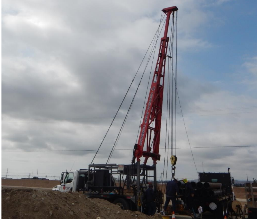
Figure 7 OH Well Replacement Program – Pump and Motor Installation
