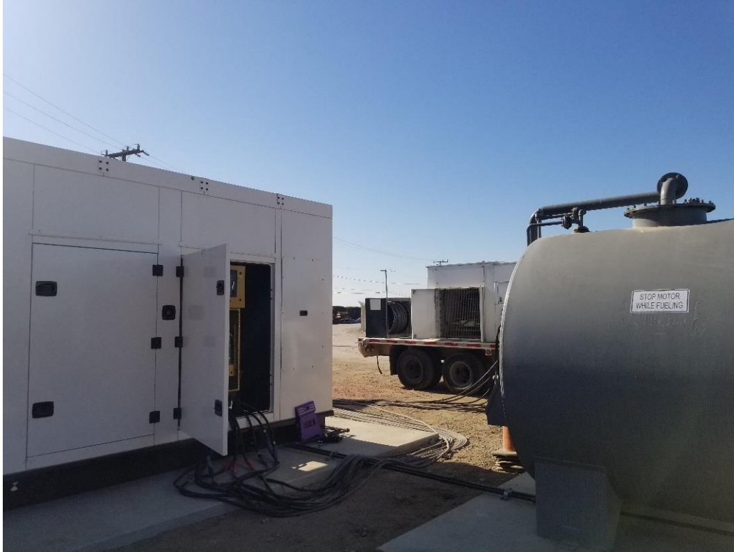
Figure 9 OH System Backup Generator Project – New Generator Load Bank Testing
