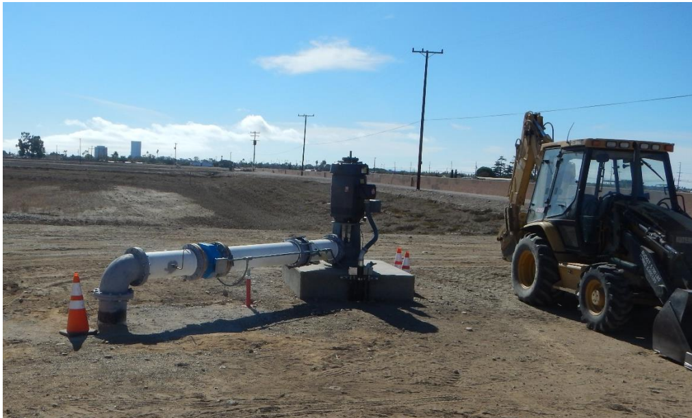
Figure 6 OH Well Replacement Program – Pump and Motor Installation
