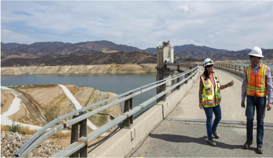
Department of Water Resources Engineer Angela Hall , left, and DWR Project Manager Jason Brabec, right, walk along the tower access bridge during this portion of a Castaic Dam Modernization Project designed to allow the facility to better withstand earthquakes' effects by among other things, wrapping piers of the dam's tower access bridge with sections of Fiber Reinforced Polymer for the first time on Oct. 4, 2021. Courtesy of Andrew Innerarity/DWR
