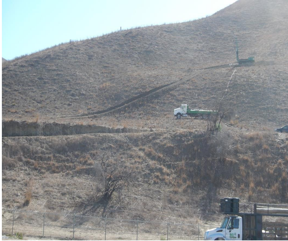
Figure 3 Freeman Diversion Rehabilitation/Fish Passage Facility Geotechnical Investigation - Installation of the Inclinometer
