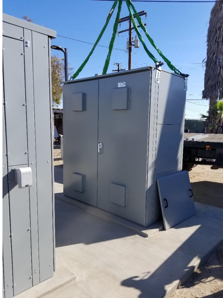
Figure 4 – OH System Backup Generator Project – Installation of ATS
