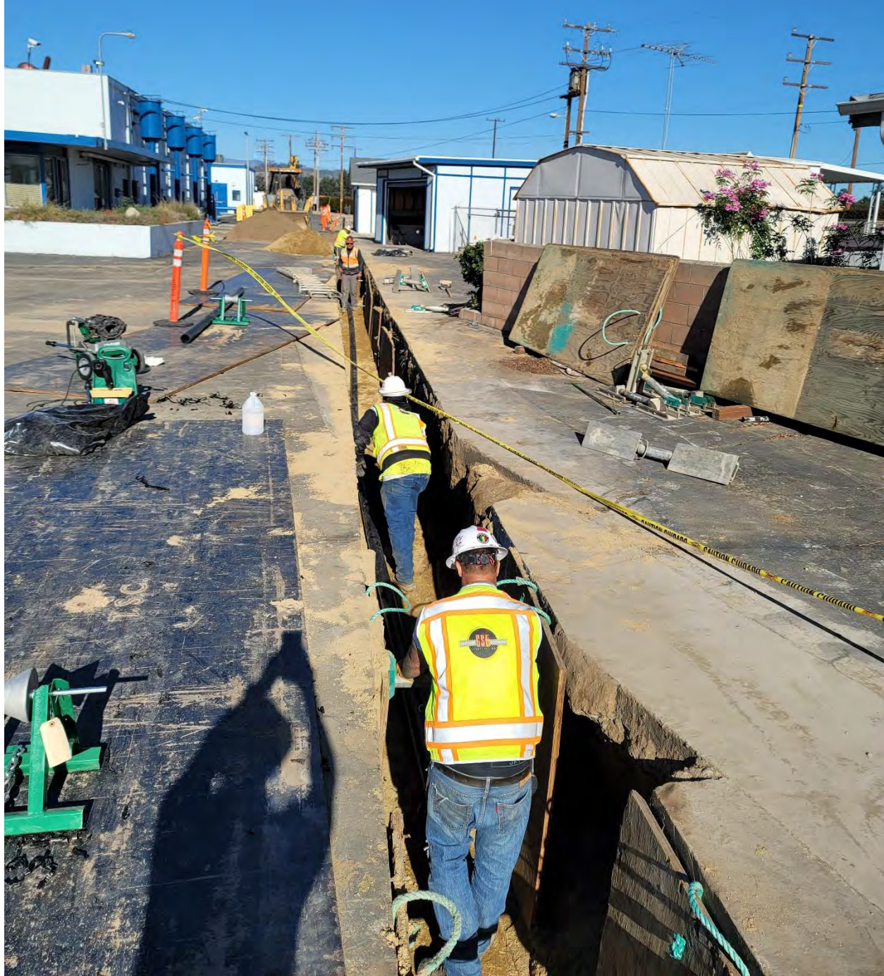
Figure 2 - Construction of 4-inch HDPE sewer line underway (photo taken Jan 27, 2022)
