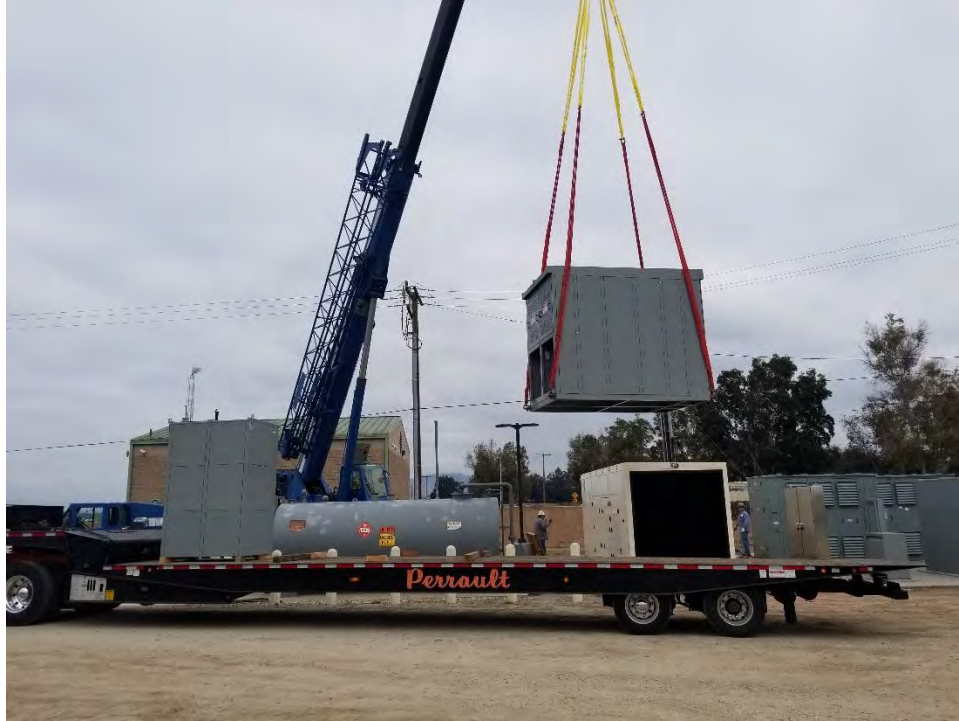
Figure 3 - OH System Backup Generator Project - Delivery of Medium Voltage Switches (photo taken Jan 19, 2022)
