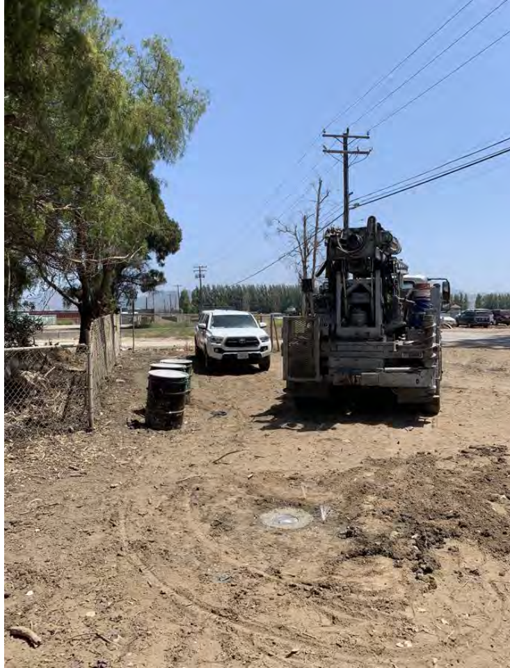
Figure 3 – Laguna Road Pipeline Project Geotechnical Boring
