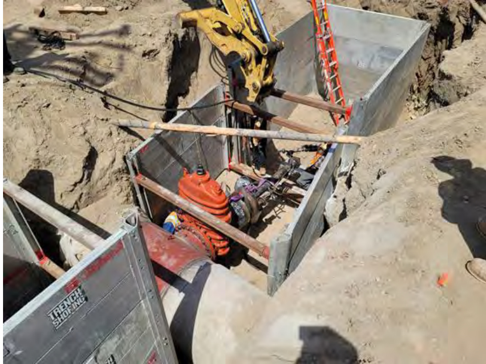
Figure 1 – Hot Tap into OH Pipeline for BWS Pipeline
