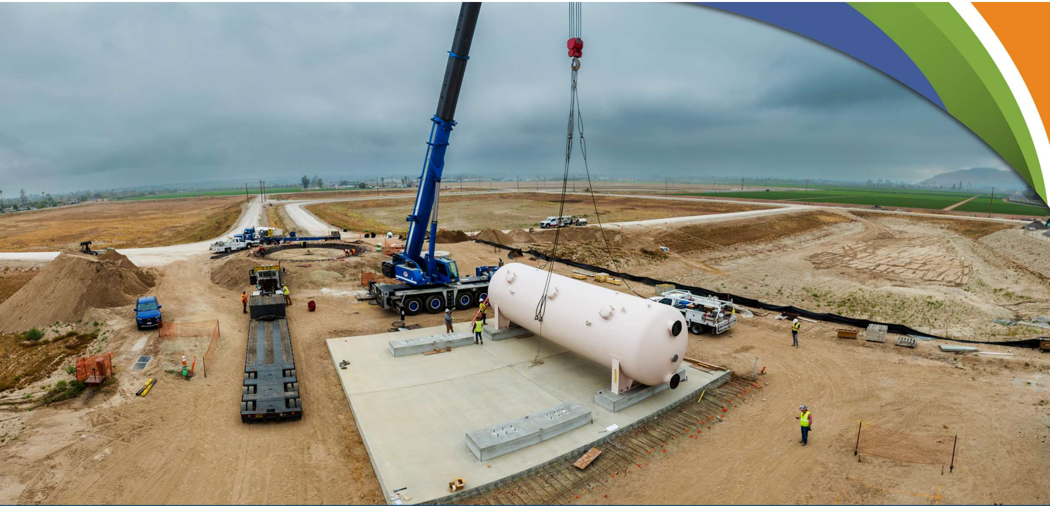
Filter Vessel Installation (June 2022)
