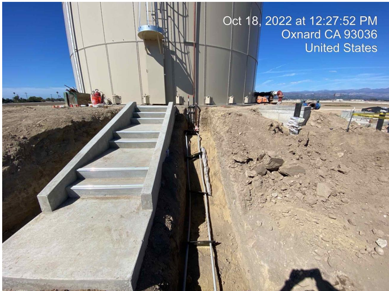
Figure 2 - 2.5" Copper Utility Water and Electrical Conduit Installation at Wash water Recovery Tank
