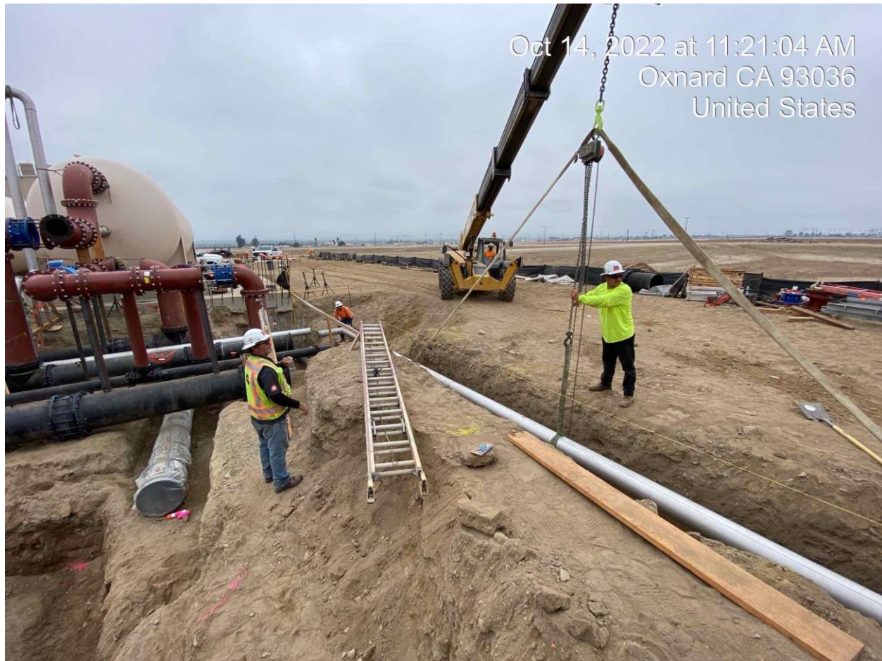
Figure 1 - 8" Welded Stainless Steel Air Supply Pipeline Installation
