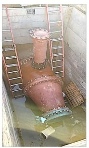
New 24" Filtered Water Connection to Existing 42" Upper Aquifer System Pipeline
