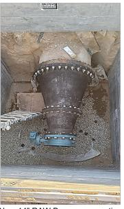
New 14" RAW Bypass connection to Existing 42" Upper Aquifer System Pipeline
