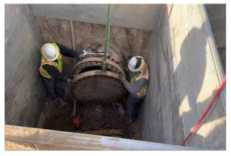
GSE Construction removing 36" blind flange from existing Upper Aquifer System manifold on October 26
