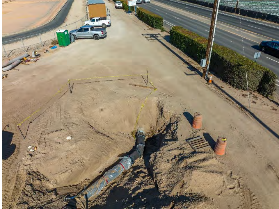
Figure 7 – RAW Pipeline Tie-In to Well 12 and 13 Manifold
