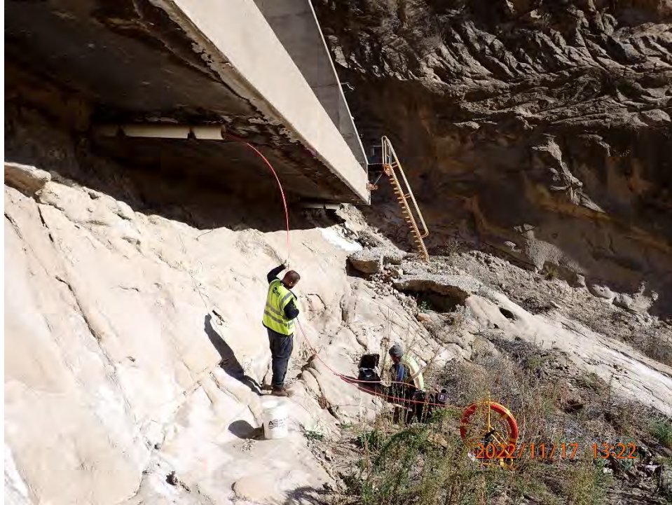
Figure 3 – Santa Felicia Dam Spillway Underdrain Inspection
