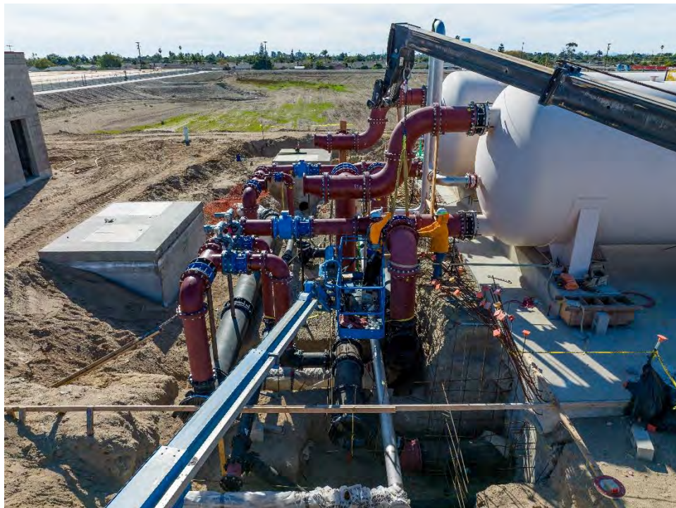
Figure 6 – Filter Face Piping Construction on November 17, 2022
