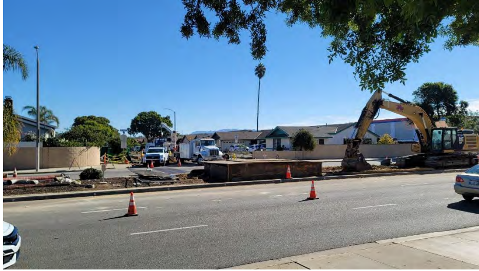
Figure 9 – Rose Avenue and La Puerta Jack & Bore Crossing under 42” OH Pipeline
