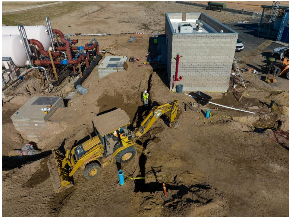
Figure 6 – Installation of 1- \frac{1}{4} " SL Pipeline and Pump Station
