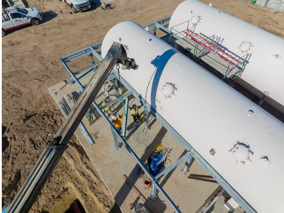
Figure 5 – Installation of Elevated Platform at Filter Vessels
