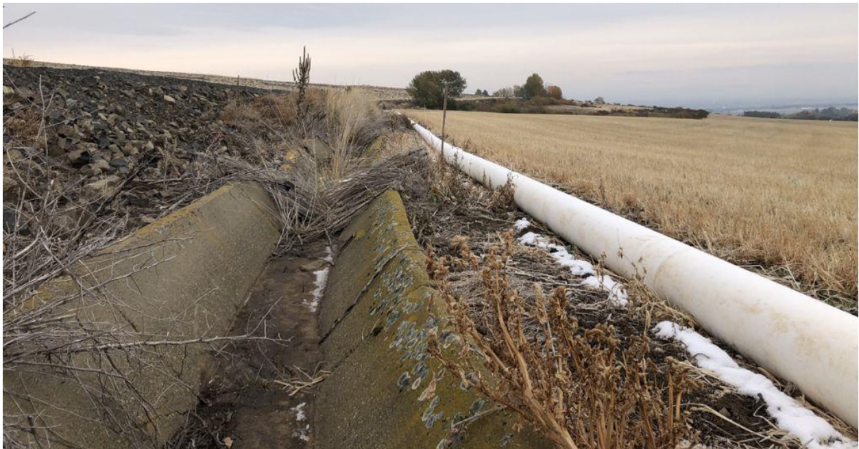
Ditching ditches: Water-saving pipes are replacing irrigation trenches, which are prone to water loss through evaporation. Photo: Nathan Gilles
