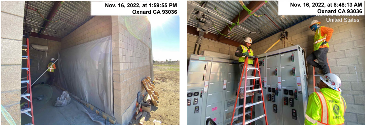
Installation of MCC in the Fe/Mn Building
