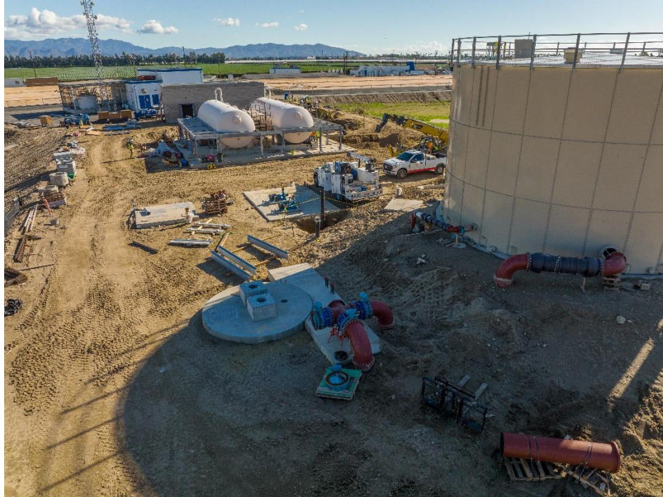
Figure 7 – Installation of above-ground piping at FD and RWW Pump Stations
