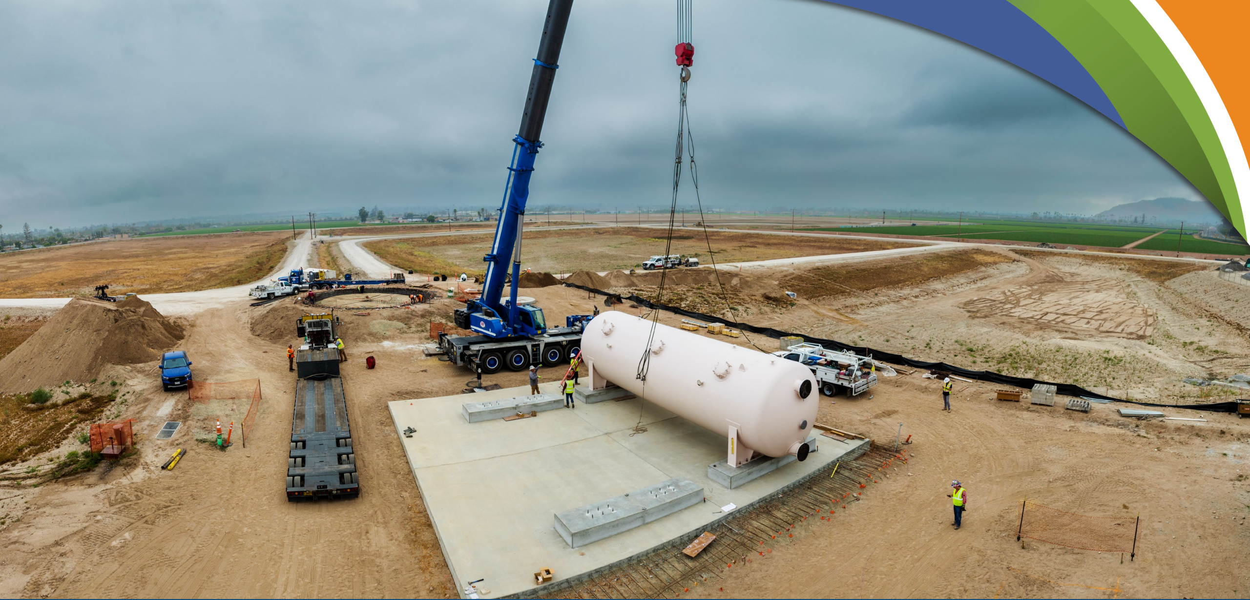
Filter Vessel Installation (June 2022)
