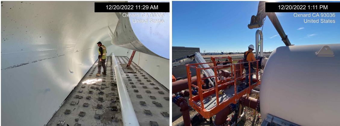
Preparing filter vessels for pressure washing and face piping for pressure testing
