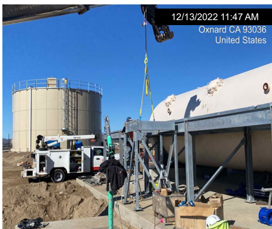
Installation of grated platforms at filter vessels
