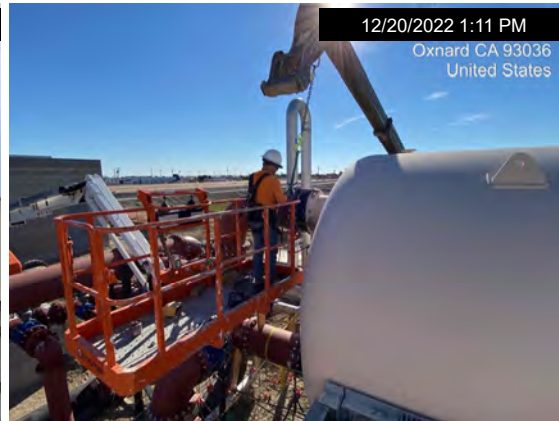
Preparing filter vessels for pressure washing and face piping for pressure testing
