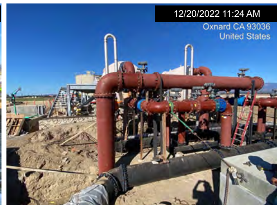
Near completion of piping at Washwater Recovery Tank and Filter Vessels
