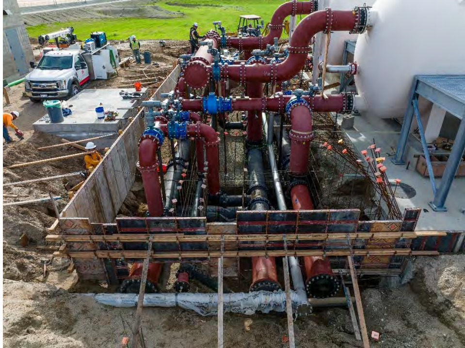
Figure 2 – Construction of Concrete Encasement and Filter Vessel Slab Formwork on January 12, 2023
