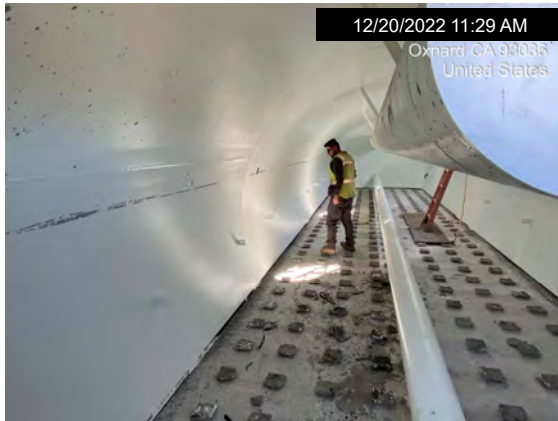
Preparing filter vessels for pressure washing and face piping for pressure testing
