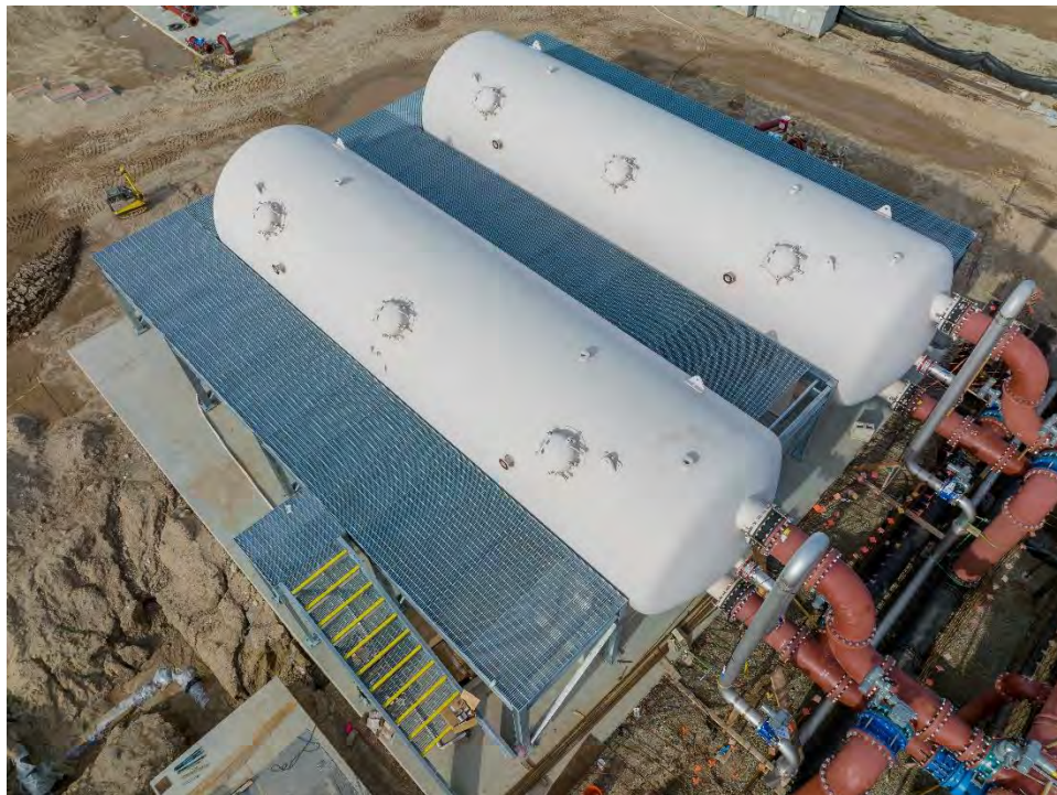
Figure 3 – Elevated Filter Vessel Platform on January 12, 2023
