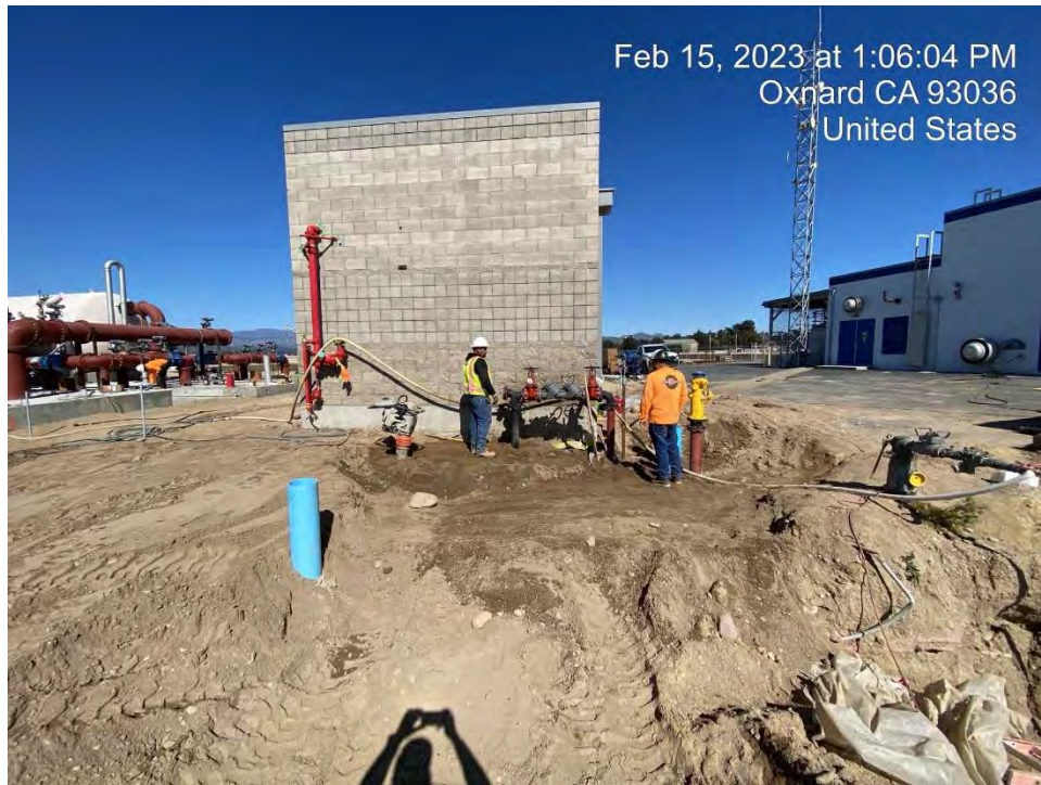
Figure 4 - Backwash Service Installation for Fire Suppression and Utility Water
