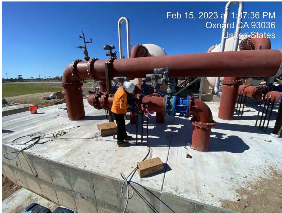
Figure 6 - Filter Vessel Face Piping Slab Complete
