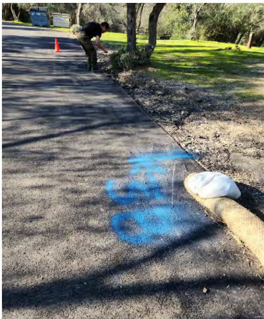
Figure 7 - Deteriorated Asphalt Area and Edge of Road Marking
