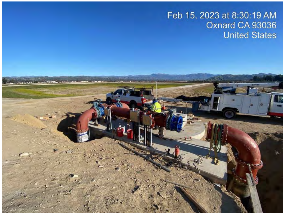
Figure 3 - Filter Drain Pump Station Installation
