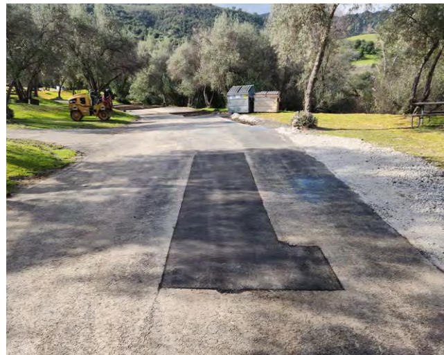
Figure 8 - Asphalt and Shoulder Backing Repair
