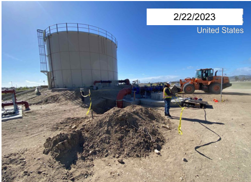
Backfill of Piping near Tank
