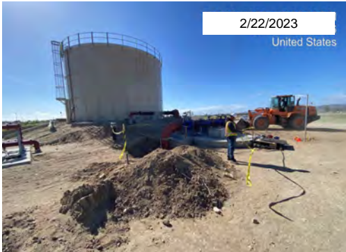
Backfill of Piping near Tank
