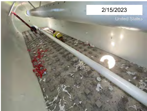
Cleaning Inside Filter Vessel in Preparation of a Soak Test
