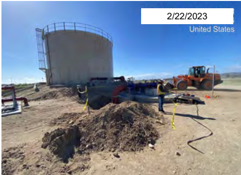
Backfill of Piping near Tank
