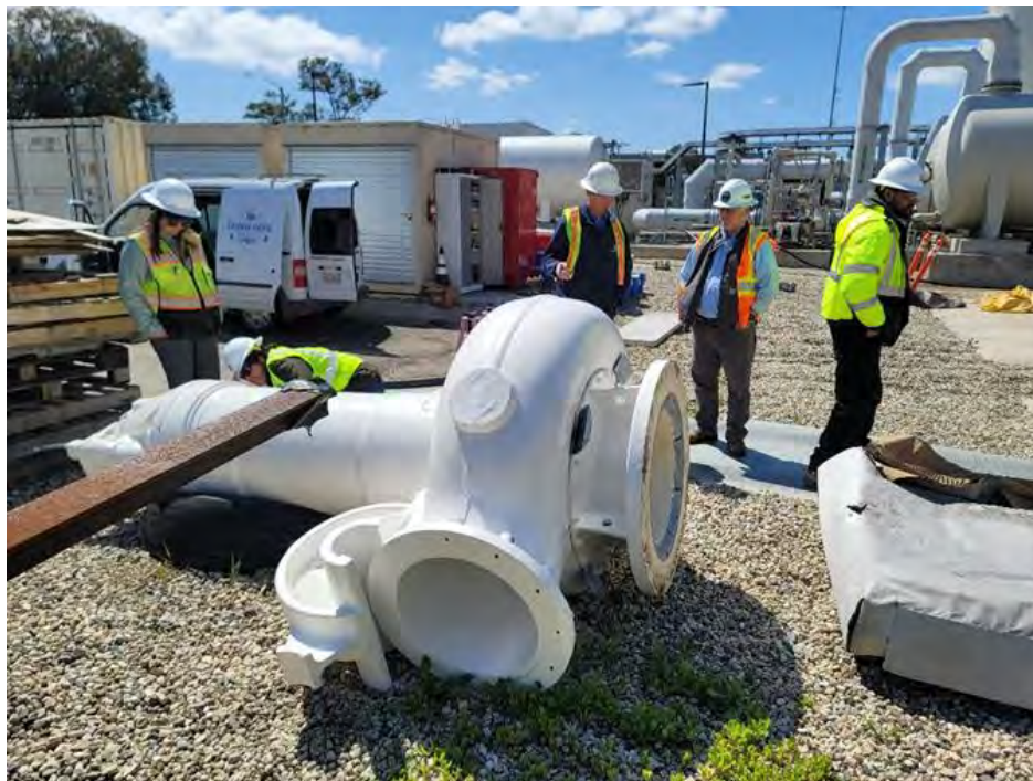
Figure 5 – Tessa Lenz, Dan Detmer and Adrian Quiroz Observing Standby Seawater Intake Pump at the Charles E Meyer Desalination Plant in Santa Barbara (23-Mar-2023)
