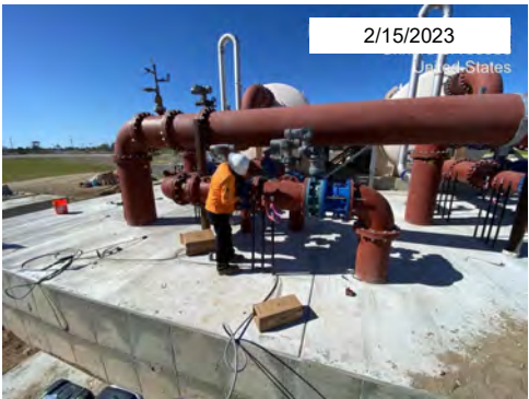
Filter Vessel Face Piping Slab Complete
