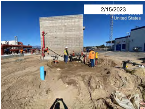
Water Service Installation for Fire Suppression and Utility Water
