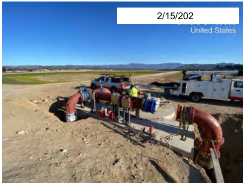
Filter Drain Pump Station Installation
