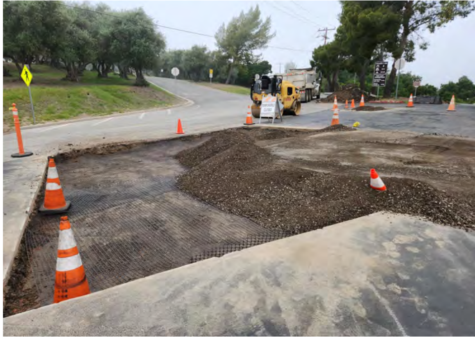
Figure 3 – Asphalt Repair at Lake Piru Recreation Area, April 24
