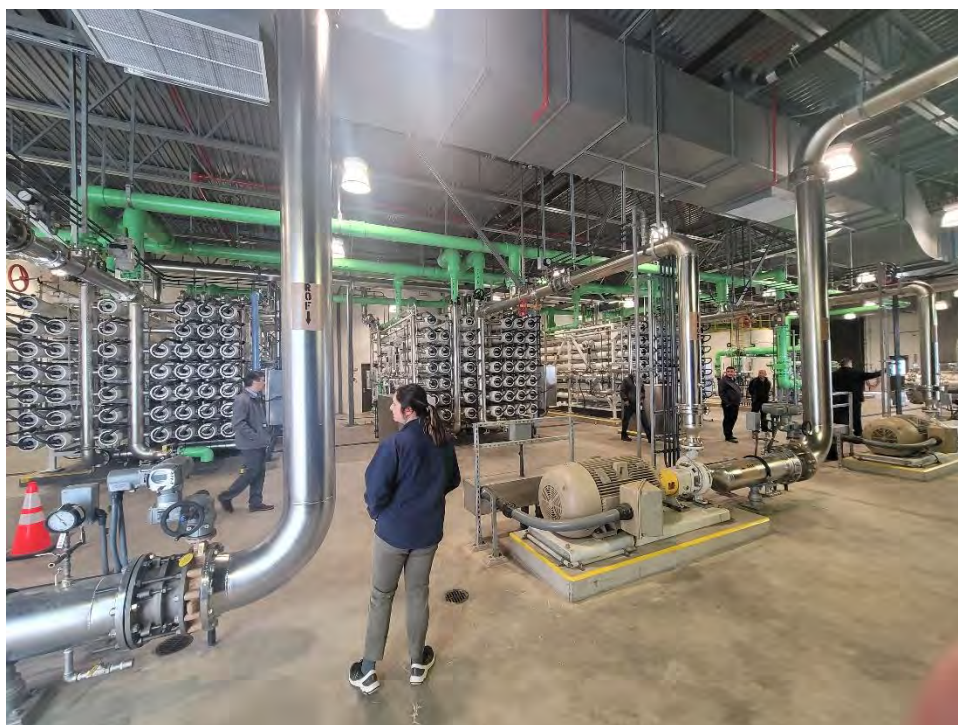
Figure 2 - Tour of the Perris II Desalter (Tessa L. shown near the primary feed pumps to the reverse osmosis treatment trains)
