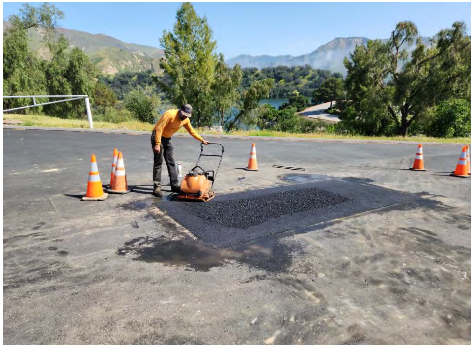
Figure 4 – Asphalt Repair at Lake Piru Recreation Area, April 24
