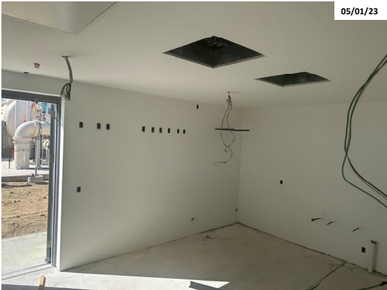
Laboratory room – dry wall installation
