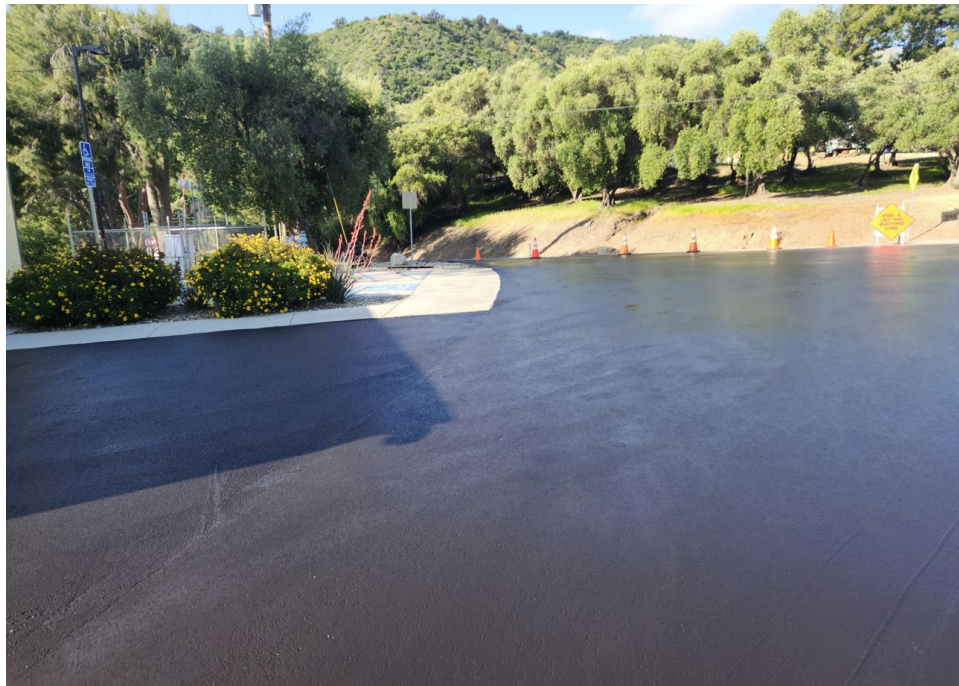
Figure 2 – Seal Coating Application at LP Recreation Area, May 11
