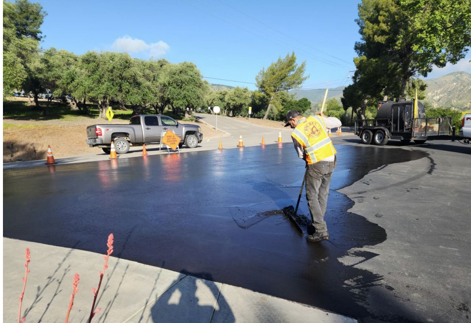
Figure 1 – Seal Coating Application at LP Recreation Area, May 11
