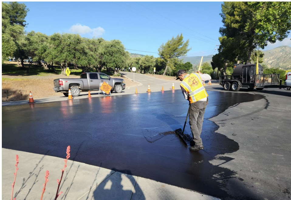
Figure 1 – Seal Coating Application at LP Recreation Area, May 11
