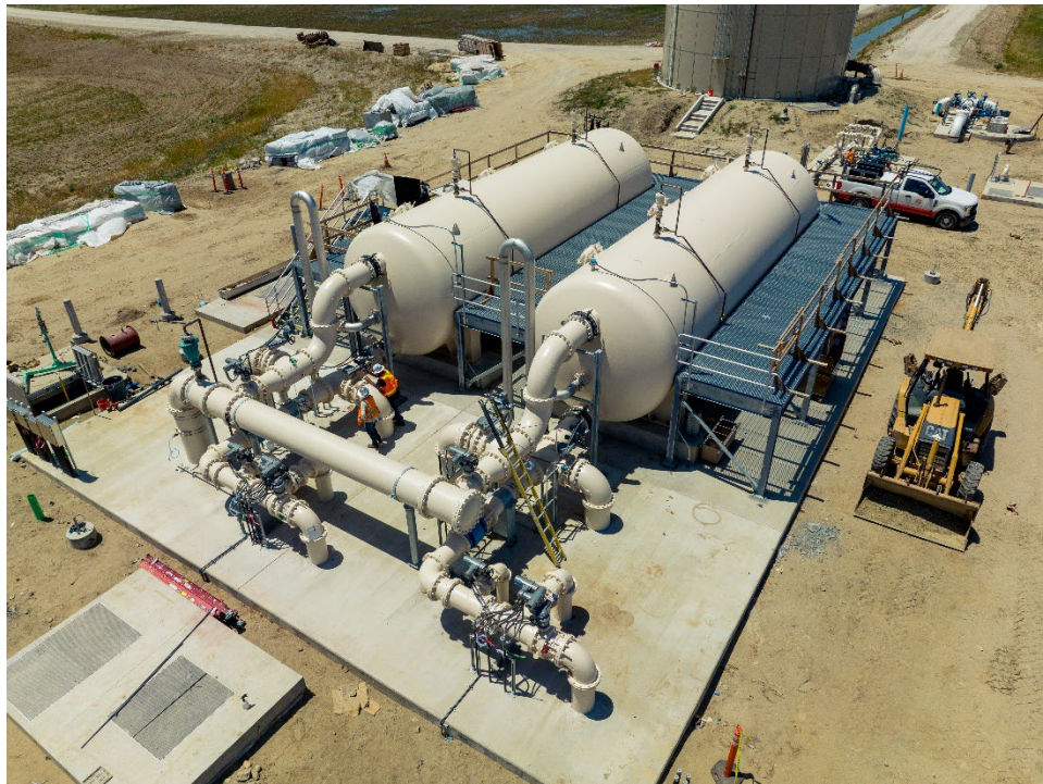
Figure 3 – Fully Coated Filter Face Piping and Filter Vessel Exterior
