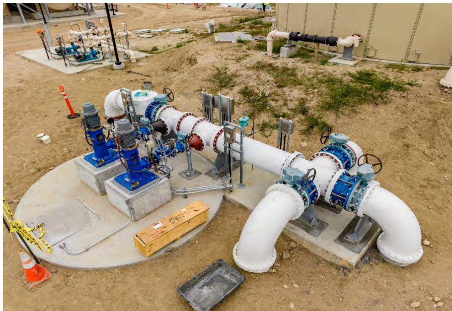
Figure 2 – Iron and Manganese Treatment Plant - Vertical Turbine Pumps at Filter Drain Pump Station
