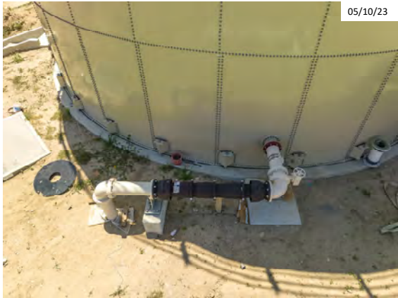
Completion of 8" Return Washwater Piping
