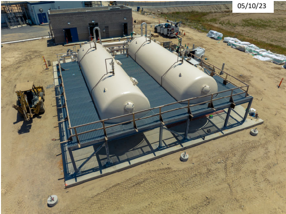
Completion of Filter Vessels Exterior and Filter Facing Piping Coating
