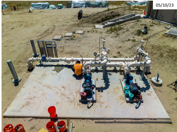
Completion of Washwater Return Pump Station
