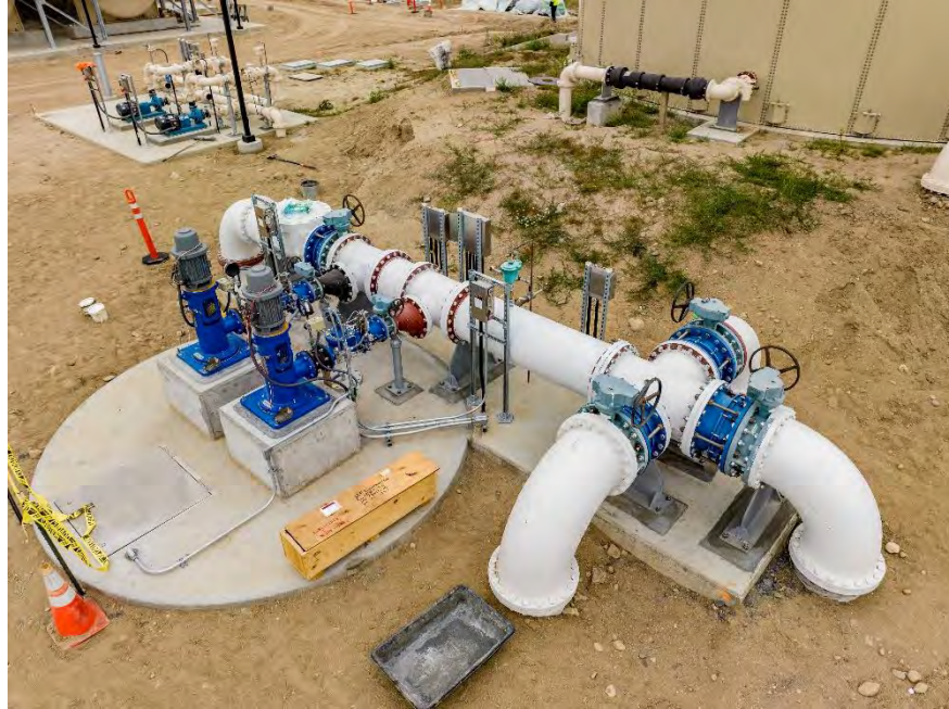
Figure 2 – Iron and Manganese Treatment Plant - Vertical Turbine Pumps at Filter Drain Pump Station
