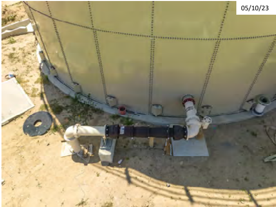
Completion of 8" Return Washwater Piping
