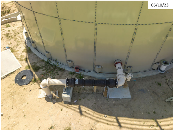
Completion of 8" Return Washwater Piping
