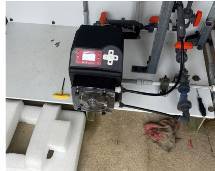
NaOCL PUMP Replacement
