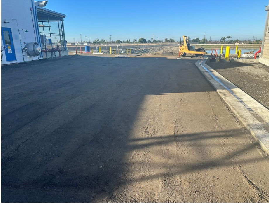
Photo 5 – Preparation for Asphalt Paving at El Rio Facility
