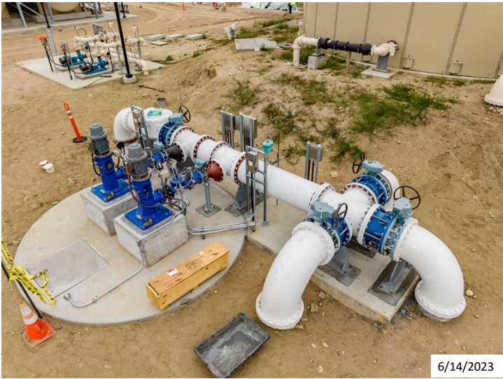
Vertical turbine pumps installed after a long delay
