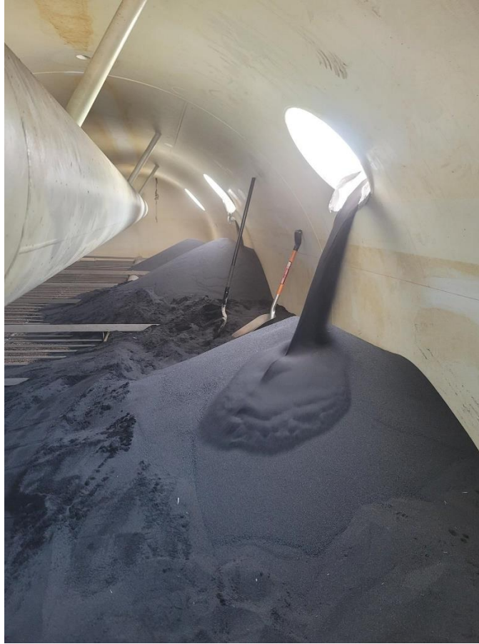
Photo 1 – Filter Media (Greensand Plus) Loading in Filter Vessel No. 2 on Sep 22
