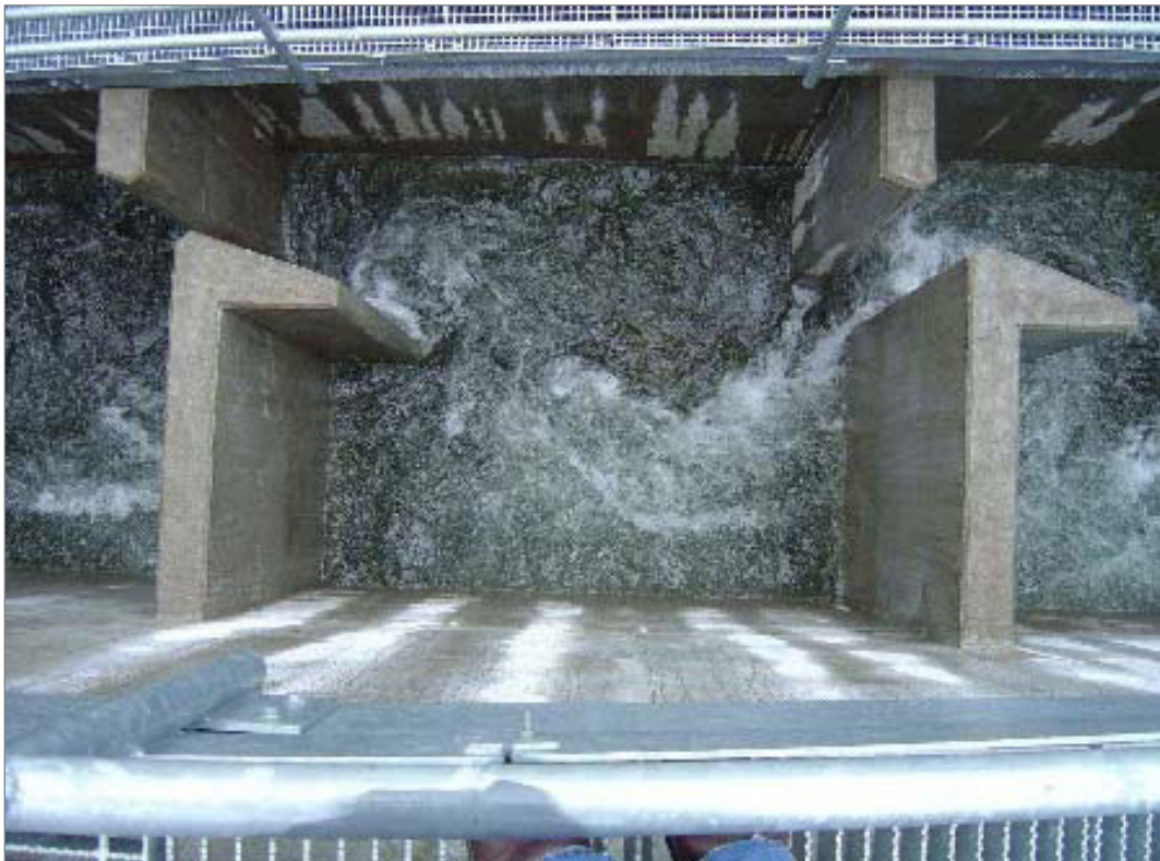
Figure 9 Typical Vertical Slot Ladder Pool
