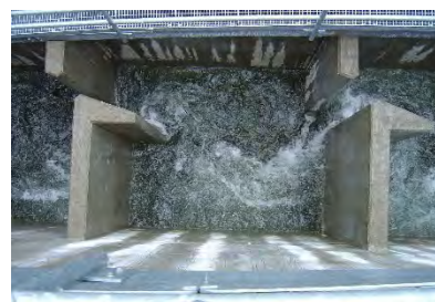
Typ. Vertical Slot Ladder Pool
