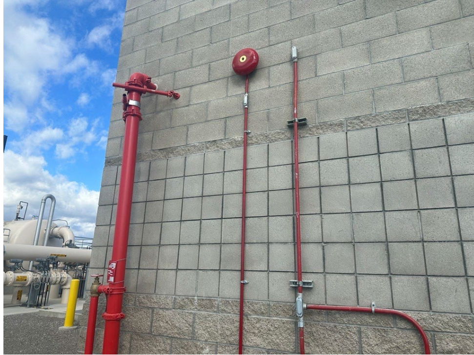
Figure 3 – Fire Alarm Bell Installation
