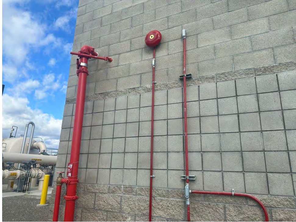
Figure 3 – Fire Alarm Bell Installation
