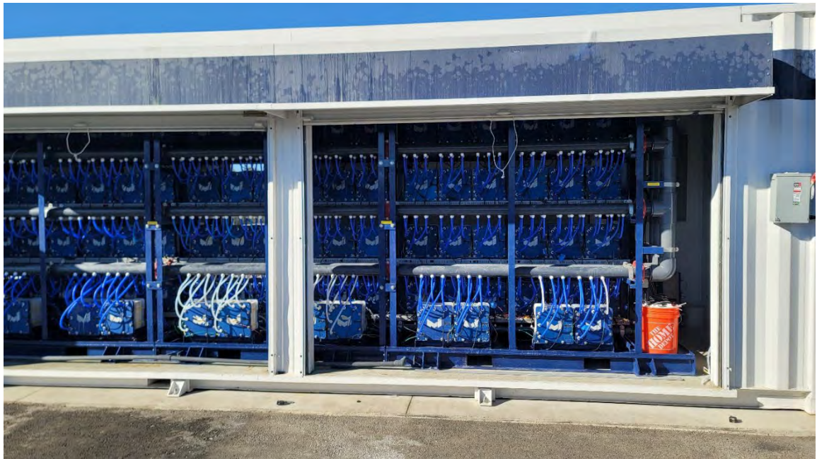
Figure 6 – “Electrochemical Nano Diffusion” System to Remove Chloride Content at the Piru Wastewater Treatment Plant (Dec 12)
