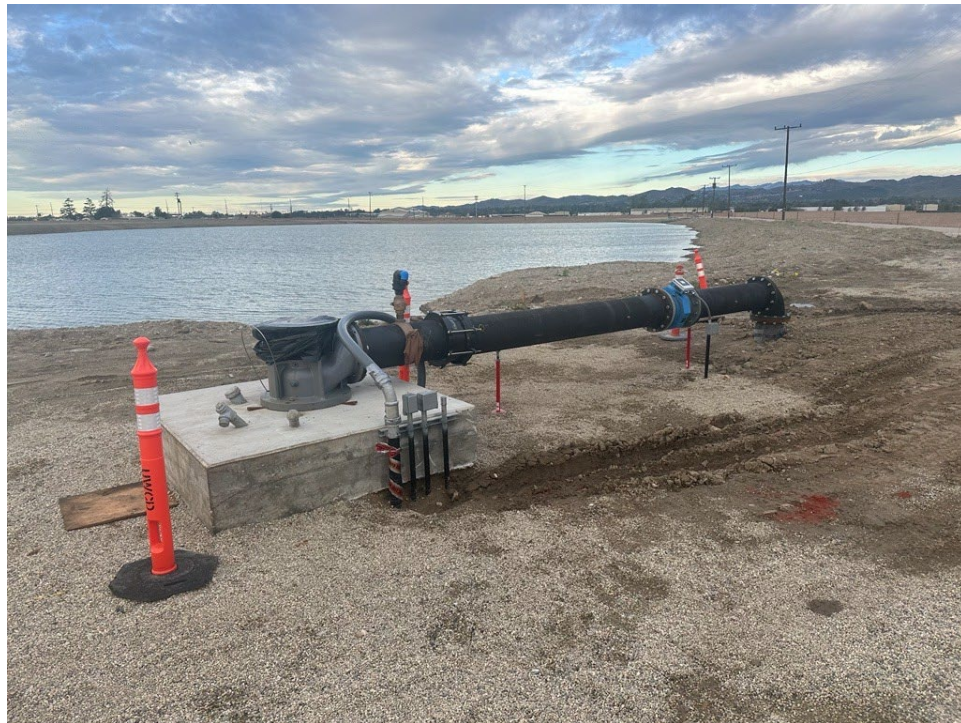
Figure 5 – New Discharge Piping at OH Well No.20
