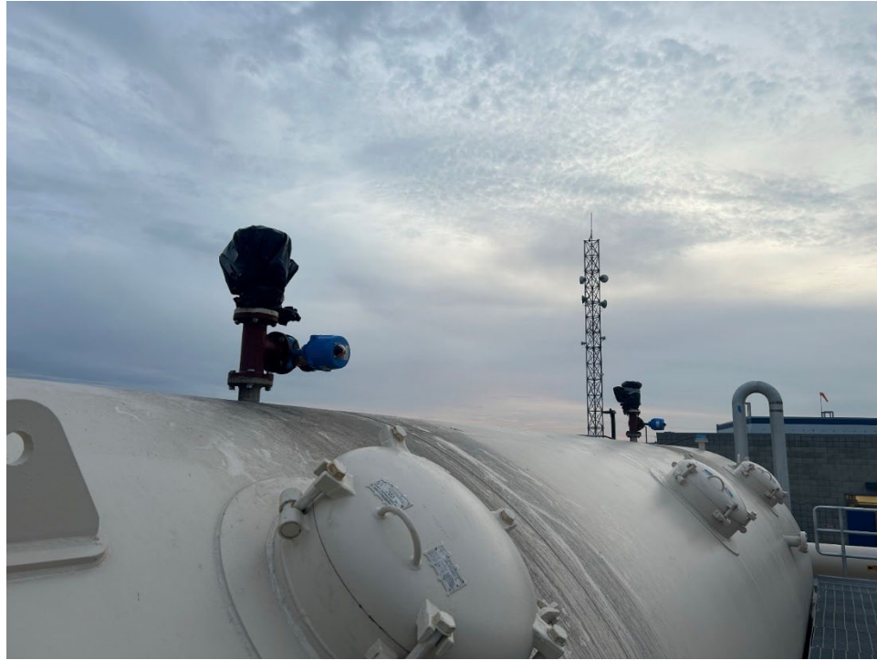
Figure 6 – Installed 3” Electrically Actuated Valves at Filter Vessel No. 2
