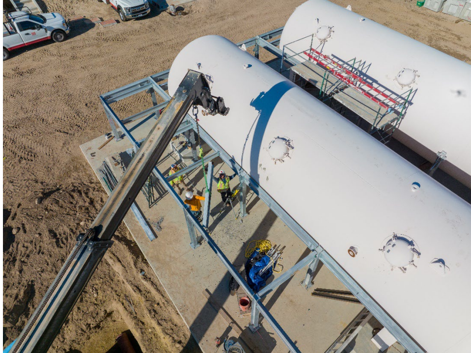
Figure 5 – Installation of Elevated Platform at Filter Vessels
