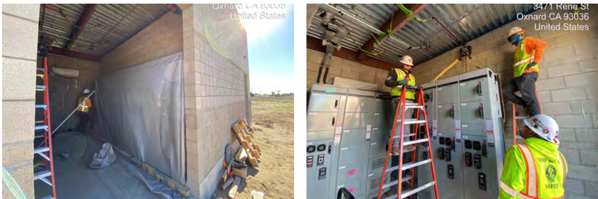
Installation of MCC in the Fe/Mn Building
