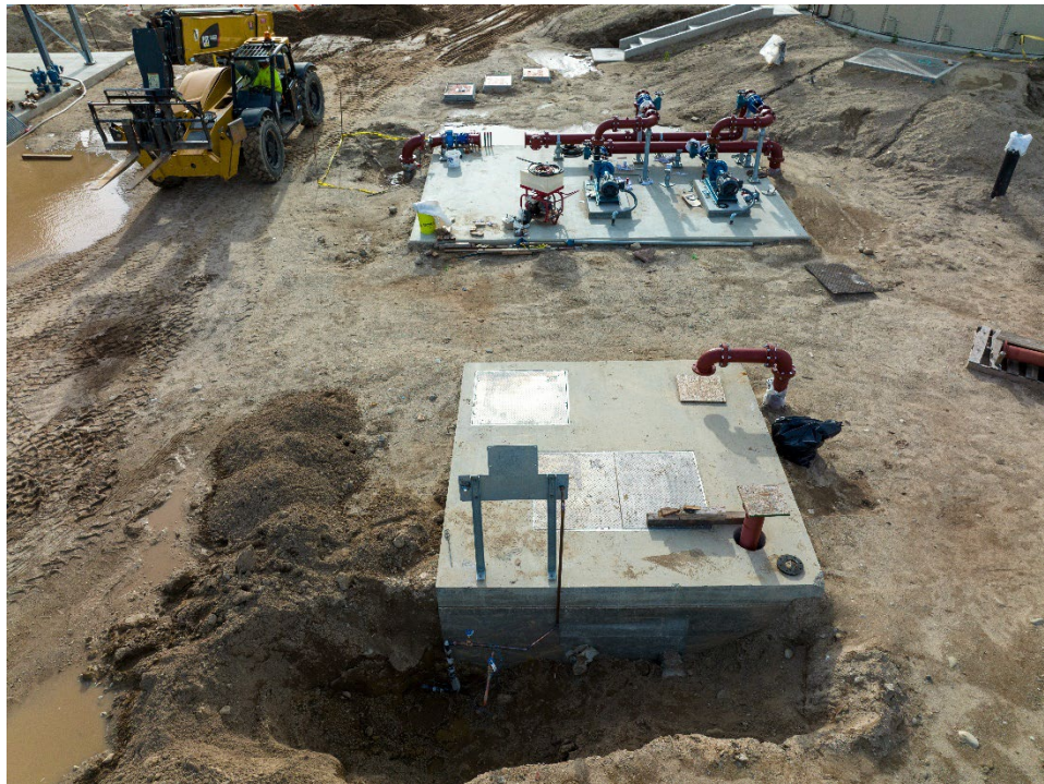
Figure 1 – Construction of Filter Drain and Washwater Return Pump Stations on January 12, 2023
