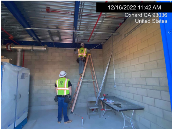
Taft installing overhead electrical conduits in electrical and blower rooms
