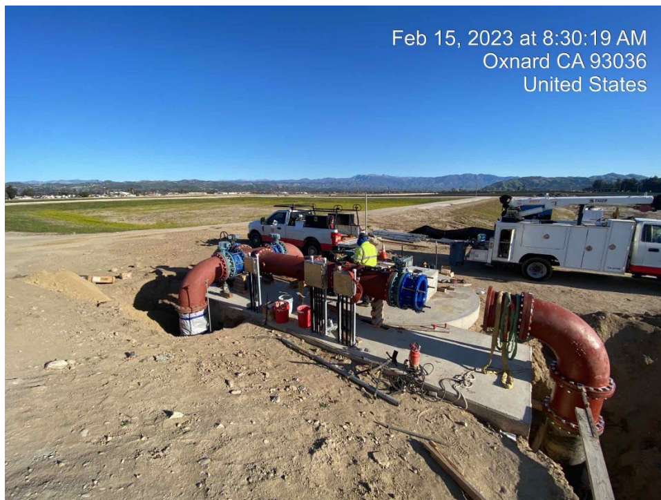
Figure 3 - Filter Drain Pump Station Installation
