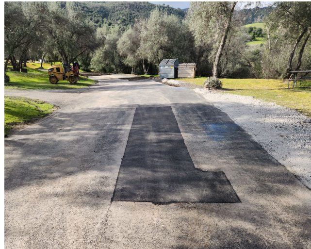
Figure 8 - Asphalt and Shoulder Backing Repair
