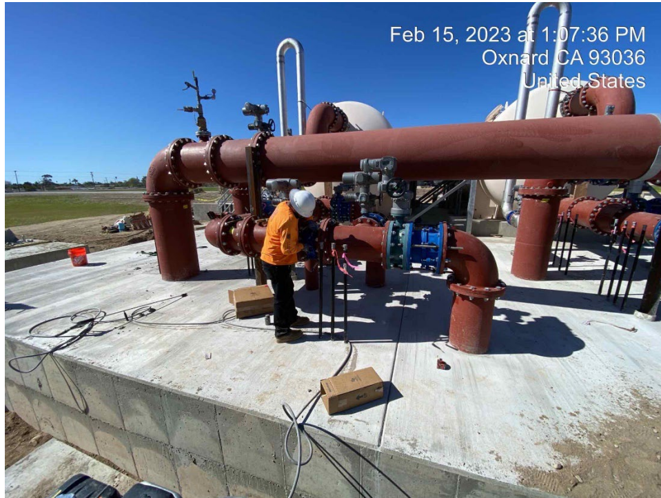
Figure 6 - Filter Vessel Face Piping Slab Complete
