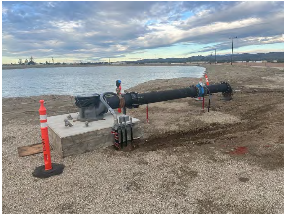
Figure 5 – New Discharge Piping at OH Well No.20
